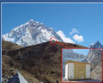
Figure 3. The CMP21 pyranometer (up) installed at the NCO-P site (down).
